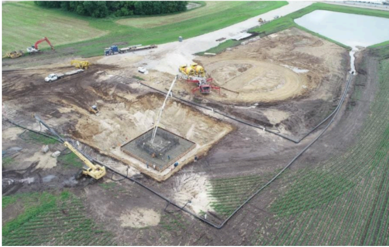
Figure 1.2a – In 2020, a dewatering activity for construction, southeast of SAA created a cone of depression and lowered the GW table below our study site. To remedy the lower level of GW access, we installed the first set of galvanized pipe in 2021. Image from NCC.
