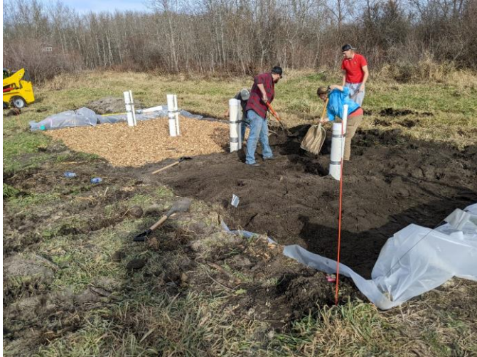
The bioreactor is covered with a soil cap during installation in November 2023.
