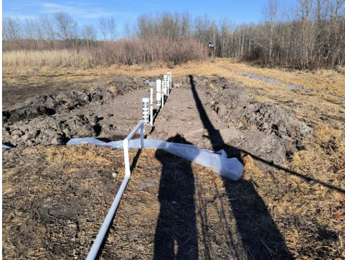
View of the bioreactor after installation in November 2023
